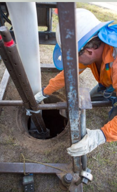
Logan Water has relined 30km of pipes in the last year
